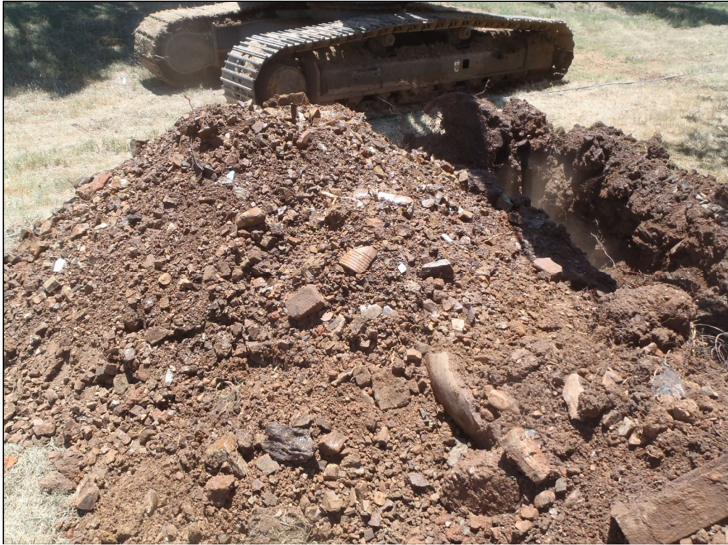
Plate 12 – Fill materials in testpit A35.
