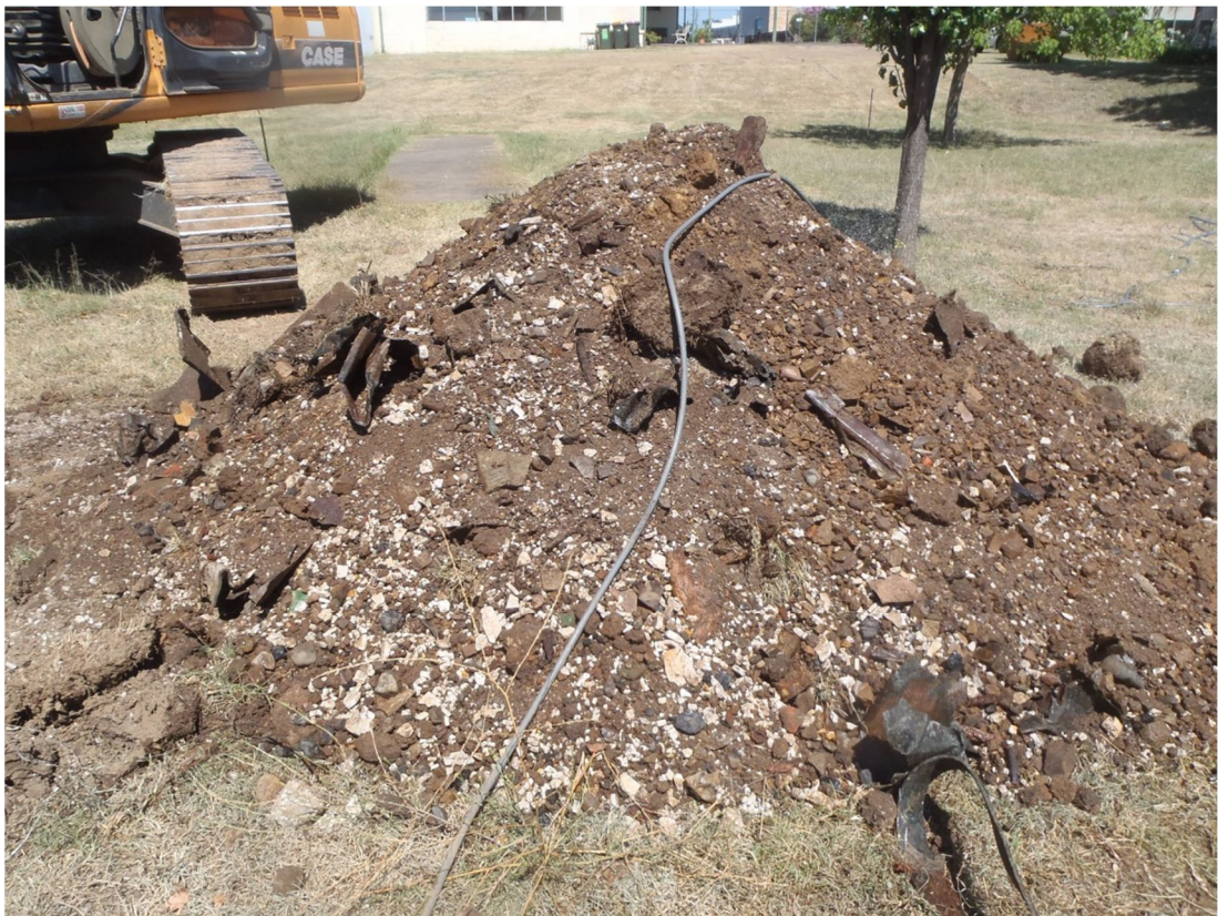
Plate 11 – Fill materials in testpit A30.
