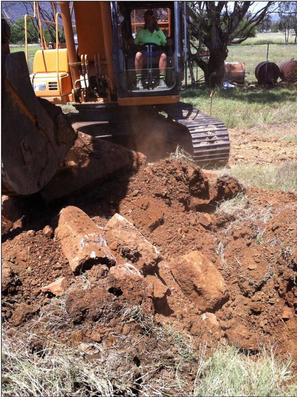
Plate 7 – Concrete footings observed in testpit A13.
