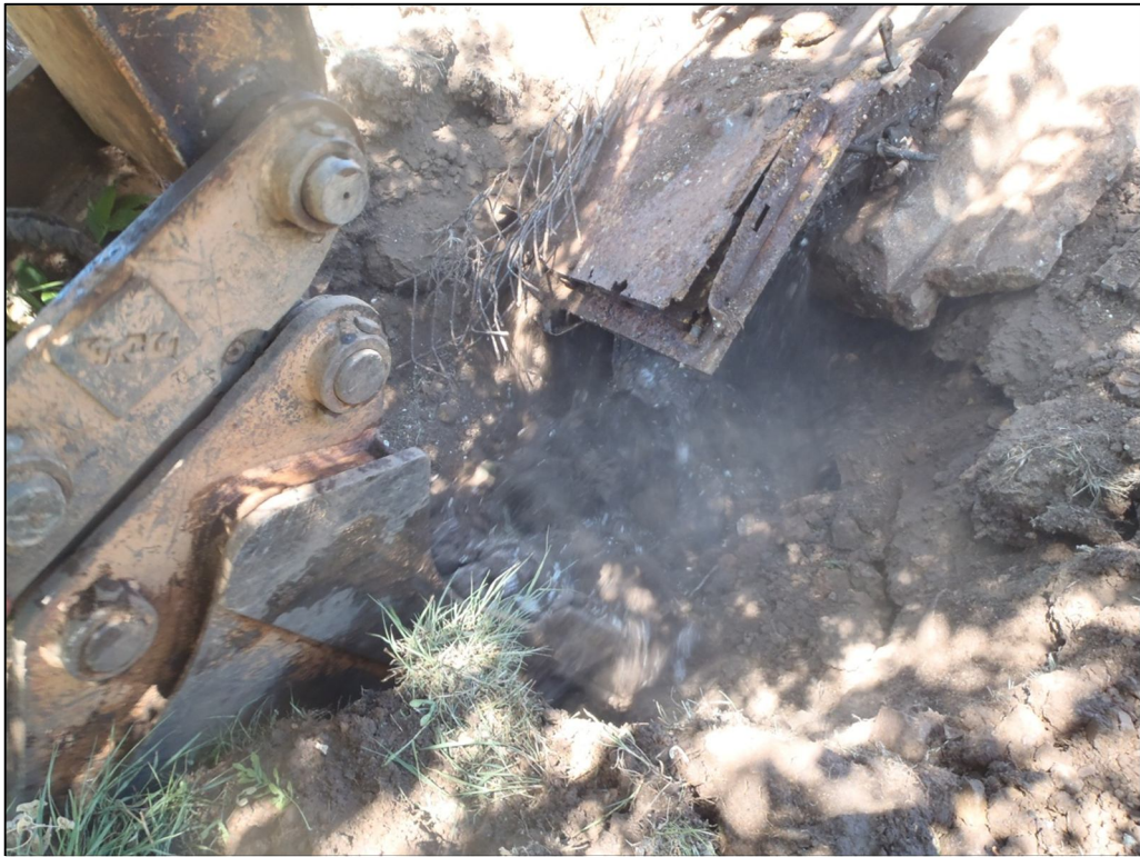
Plate 10 – Fill material in testpit A25.
